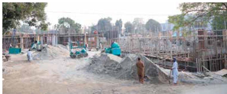
Construction of the new hostel in progress
